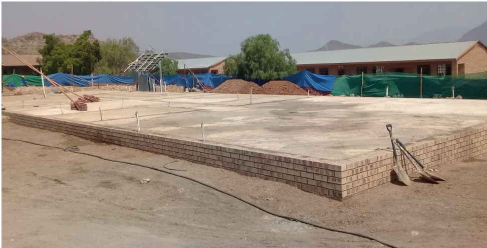
Construction site near Twickenham Mine
