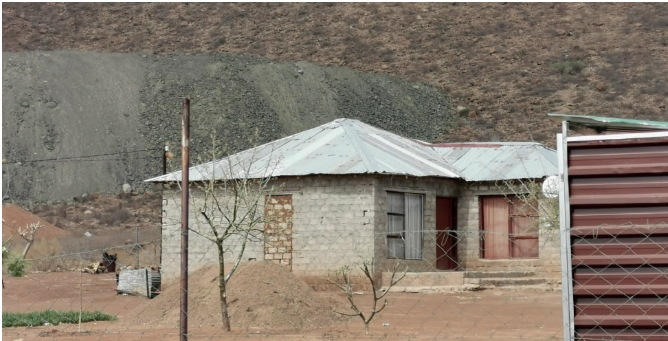
Houses on dirt roads with no water reticulation near Sefateng Mine
